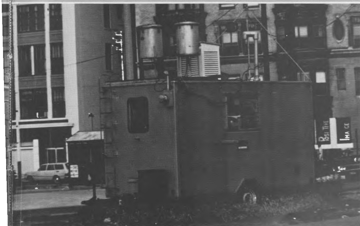
OLD MONITORING STATION
